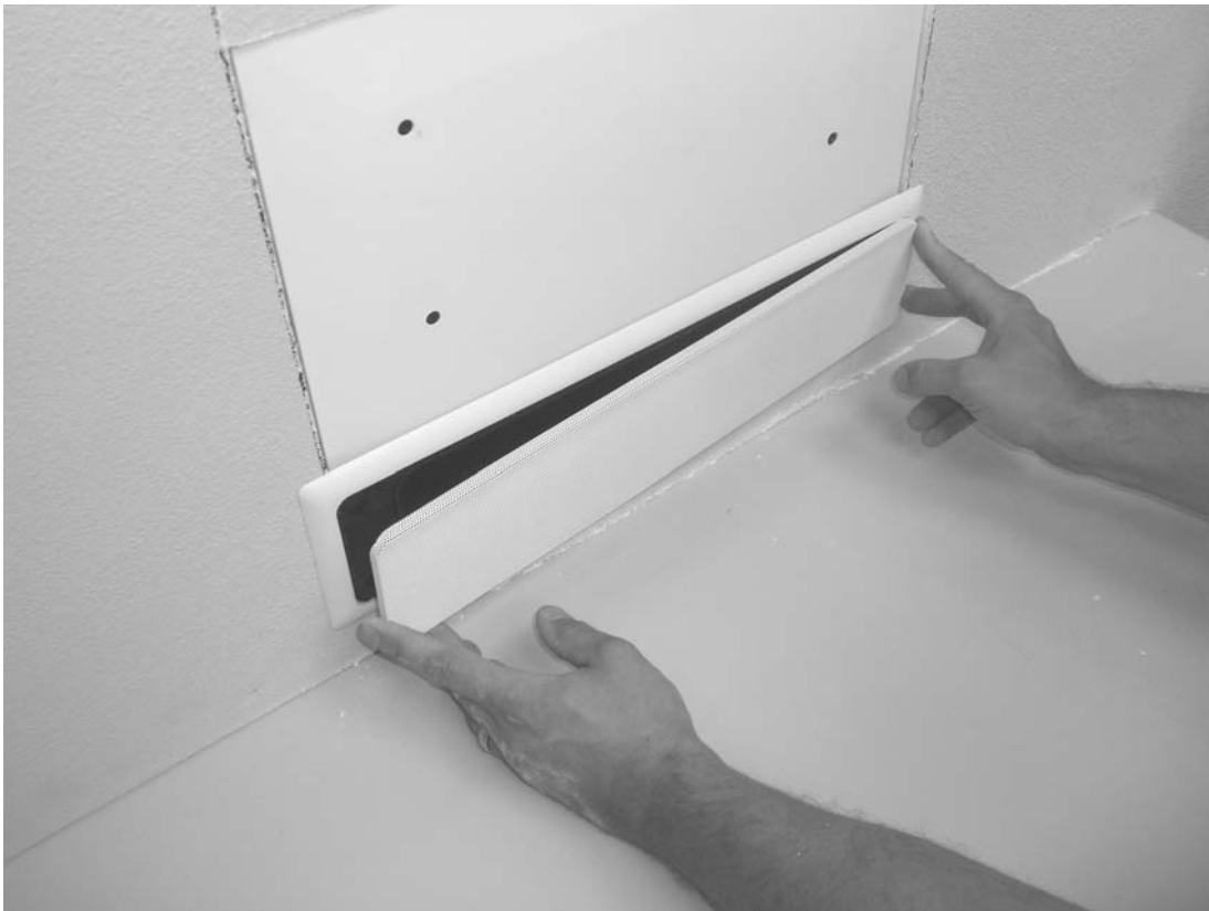
Figure 22: Metal Insert Installation
