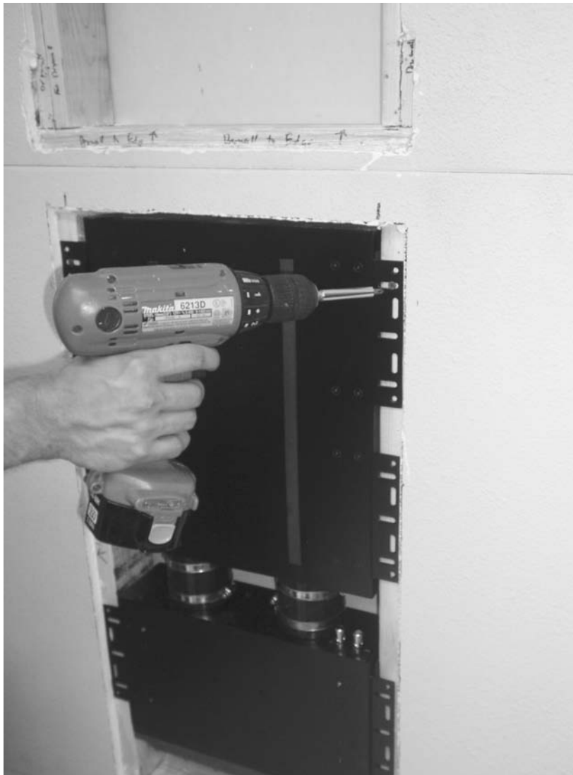
Figure 31: Secure Subwoofer
