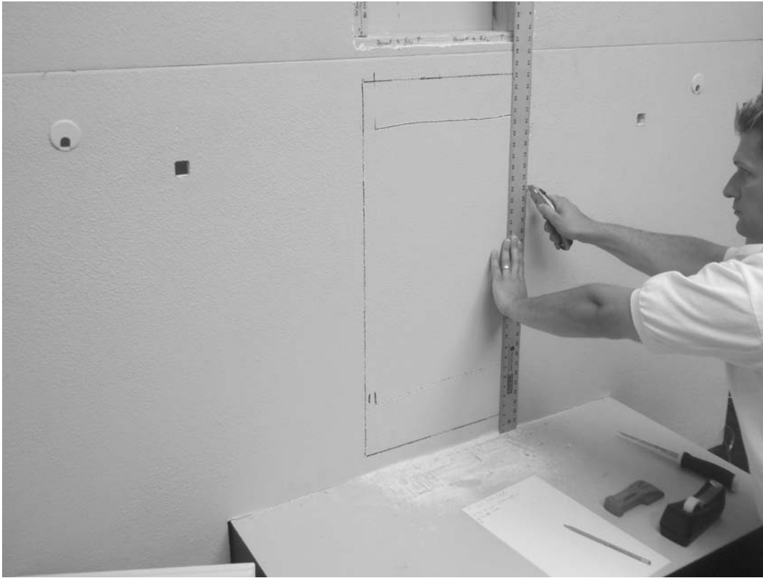
Figures 40a and 40b: Drywall Removal
