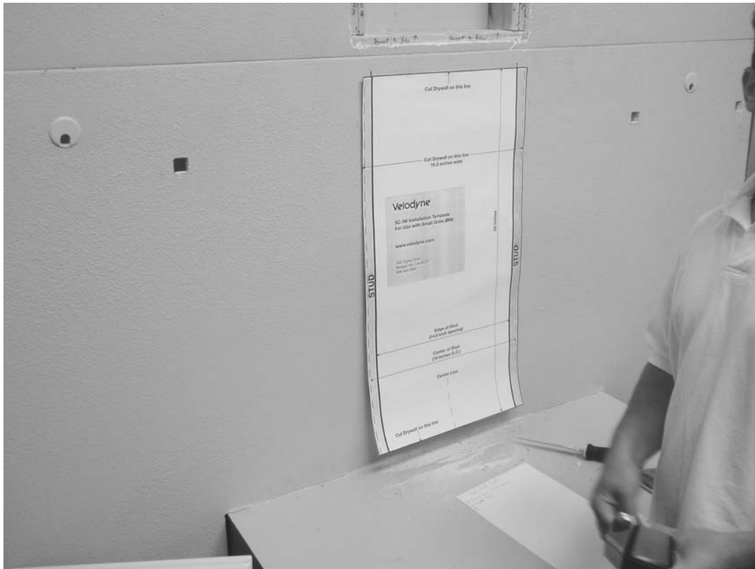
Figure 39: Cut Out Drywall
