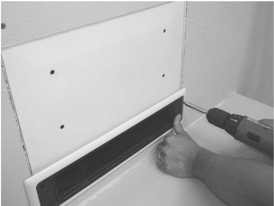
Figures 35a and 35b: Designer Grille Installation
