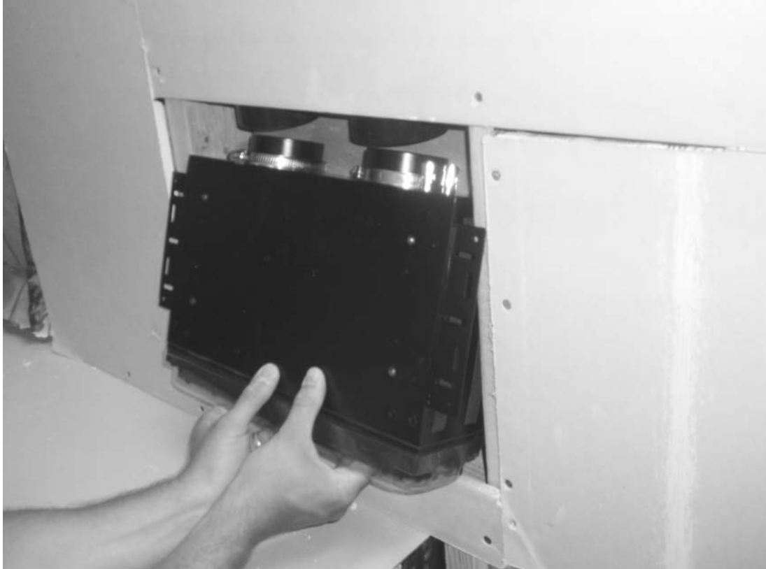
Figure 7: Driver Module Installation
