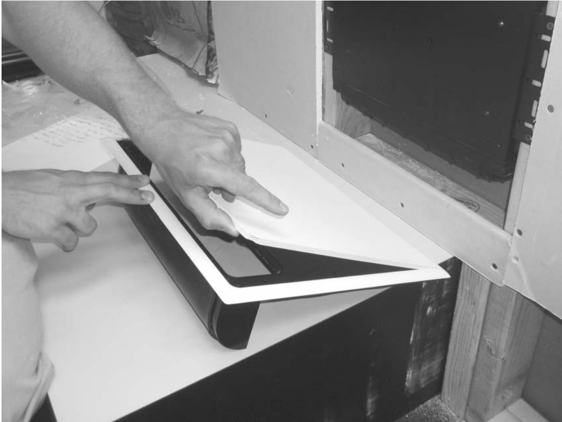
Figure 49: Metal Grille Insert Removal
