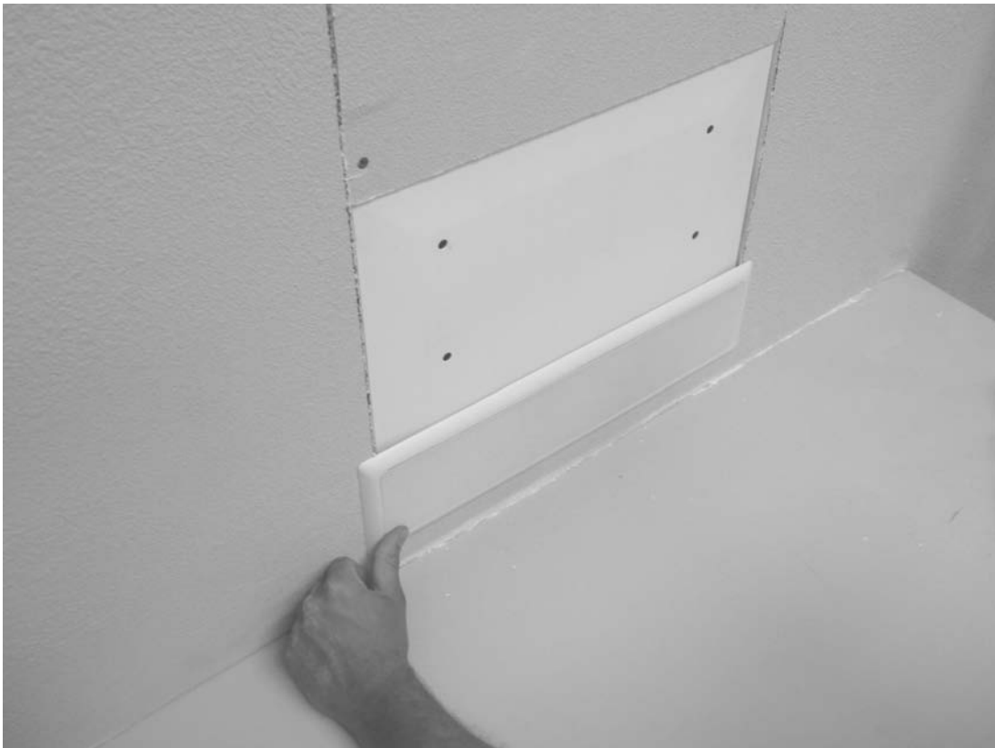
Figure 37: Finished Grille Installation
