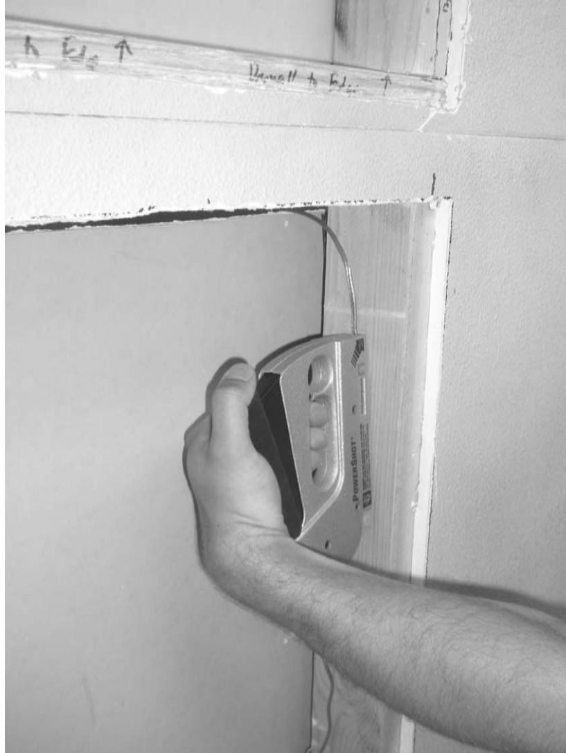
Figure 41: Speaker Wire Installation
