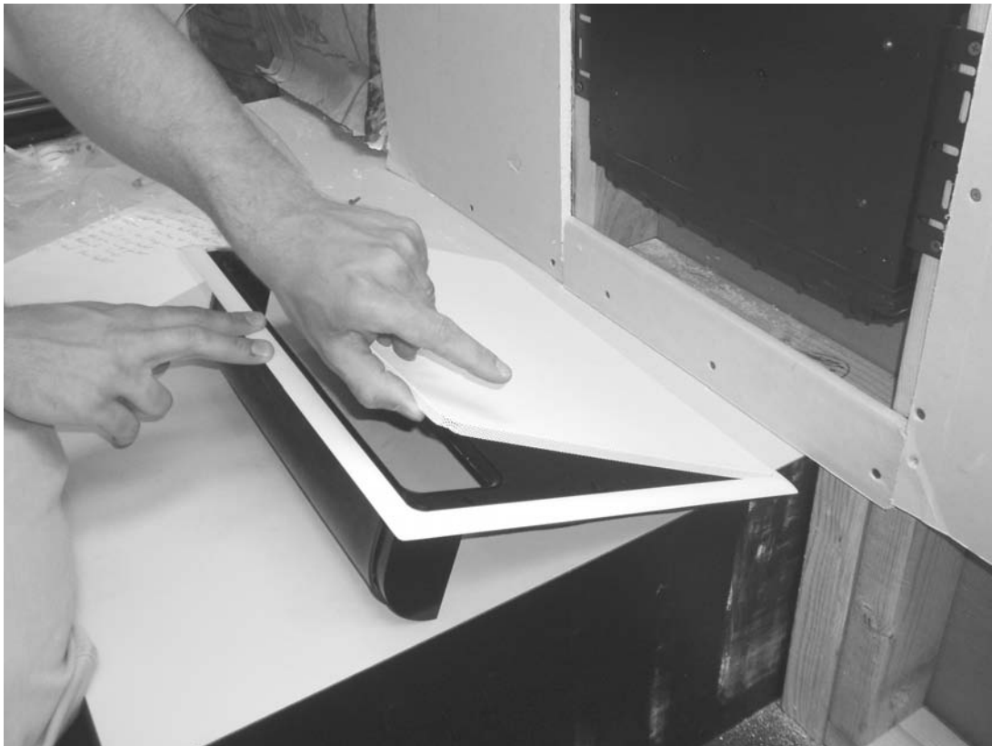
Figure 8: Metal Grille Insert Removal
