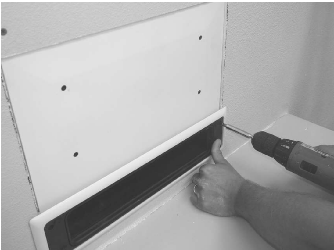
Figures 21a and 21b: Designer Grille Installation
