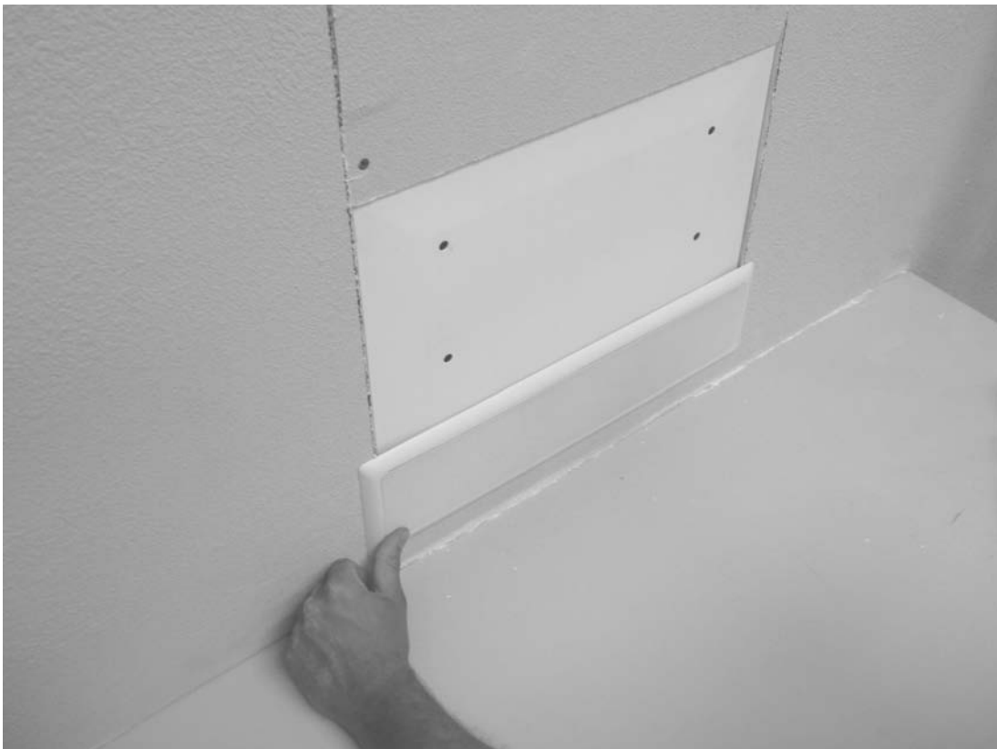
Figure 23: Finished Grille Installation
