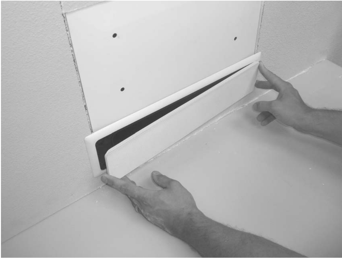
Figure 36: Metal Insert Installation
